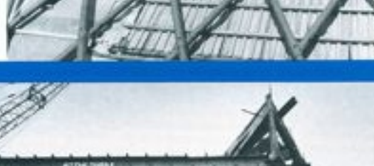
A lamella steel pipe dome crowns the General Electric Company Pavilion
