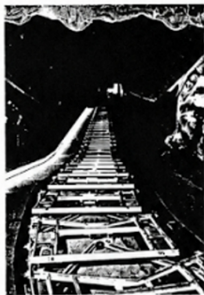
Fig. 3—A service walkway parallels the entire length of the track. This walkway is automatically lighted in case of emergency, as shown in this photograph taken during construction. Cardboard dust shields, used temporarily during the construction period, appear over the continuous center opening of the track.
