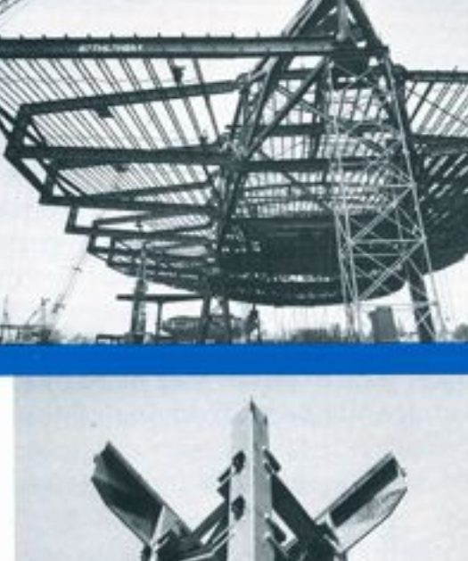
A lamella steel pipe dome crowns the General Electric Company Pavilion
