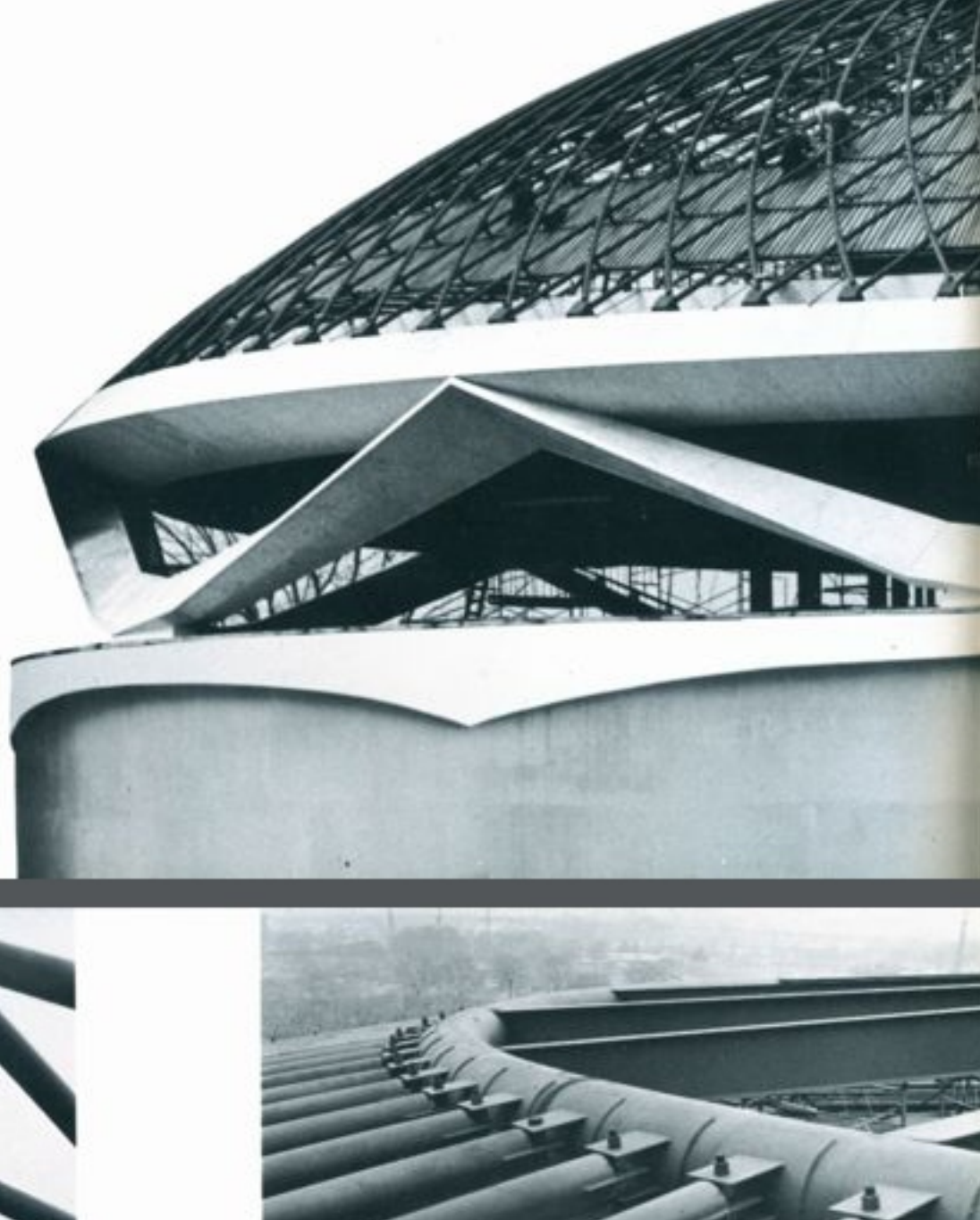
This is basically a round structure with an open circular center well, topped with a unique lamella pipe dome springing from a compression ring girder at the third level. The most unusual functional feature is a circular, rotating section, mounted on the steelwork at the second level, permitting the six theaters to rotate to each of six fixed stages. The exterior wall of the theaters is exposed to view under the deep overhang of the dome roof. The over-all effect is that of a sparkling carousel, its motion simulated by the spiraling pipe members of the dome.
