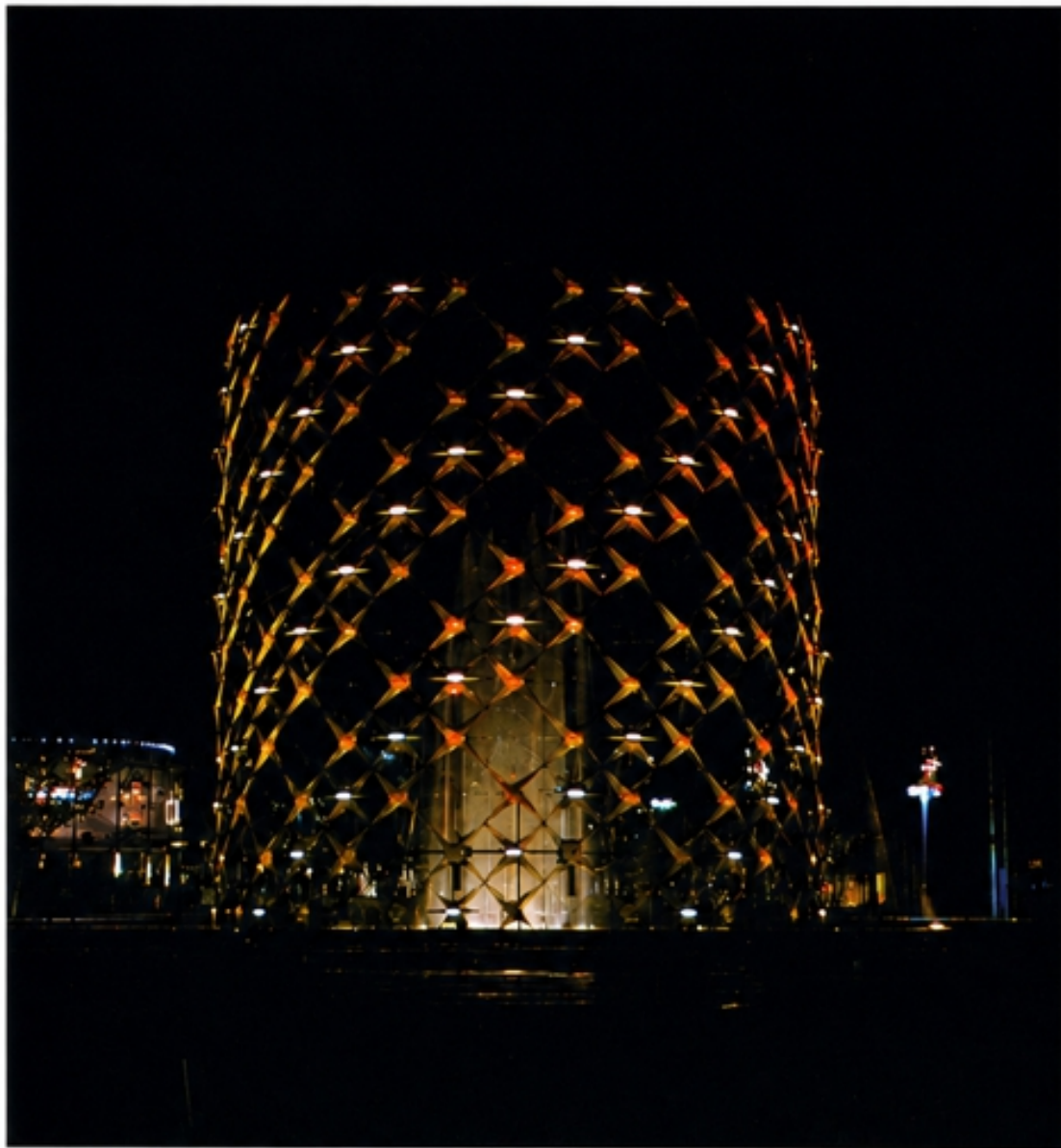
ASTRAL FOUNTAIN is the Fair's second largest. It combines a 60-ft high by 60-ft diameter rotating structure, rotating around a 70-ft high central water column, set in a 140-ft diameter pool, and colorfully illuminated at night. Lighting details are shown at left.
