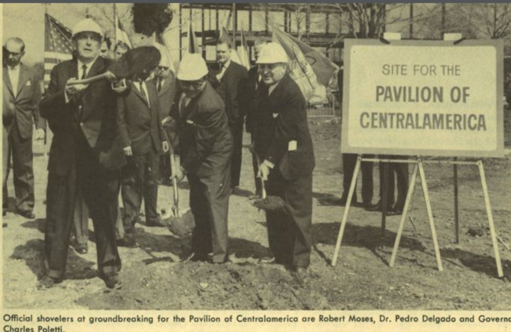
Official shovelers at groundbreaking for the Pavilion of Centralamerica are Robert Moses, Dr. Pedro Delgado and Governor Charles Poletti.
