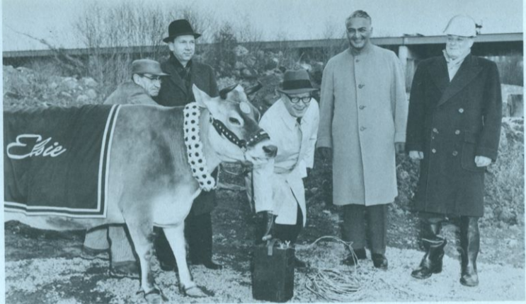
With Elsie, the Borden Cow, and her keeper, supervising, Edward Burdick pushes a plunger which blasted for the start of construction on the Better Living Building. Watching are (left to right) William Ewen, director of advertising for Borden; Martin Stone, director of the Fair's Industrial Section; J. P. Van Raalte, chairman of the board for Thompson-Starrett Construction Co., Inc.
