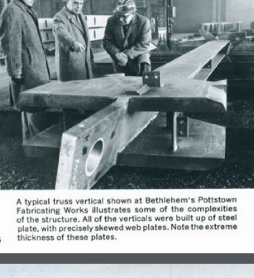
A typical truss structure at Bethlehem's Pottstown Fabricating Works illustrates some of the complexities of the structure. All of the verticals were built up of steel plate, with precisely skewed web plates. Note the extreme thickness of these plates.
