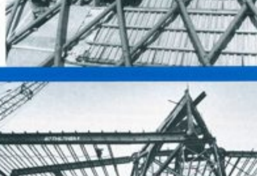
A lamella steel pipe dome crowns the General Electric Company Pavilion
